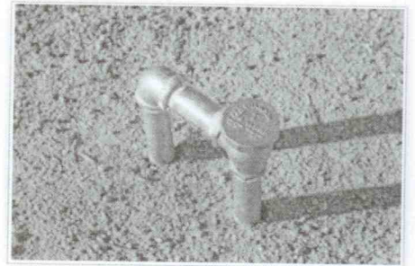
AVB - Atmospheric Vacuum Breaker
